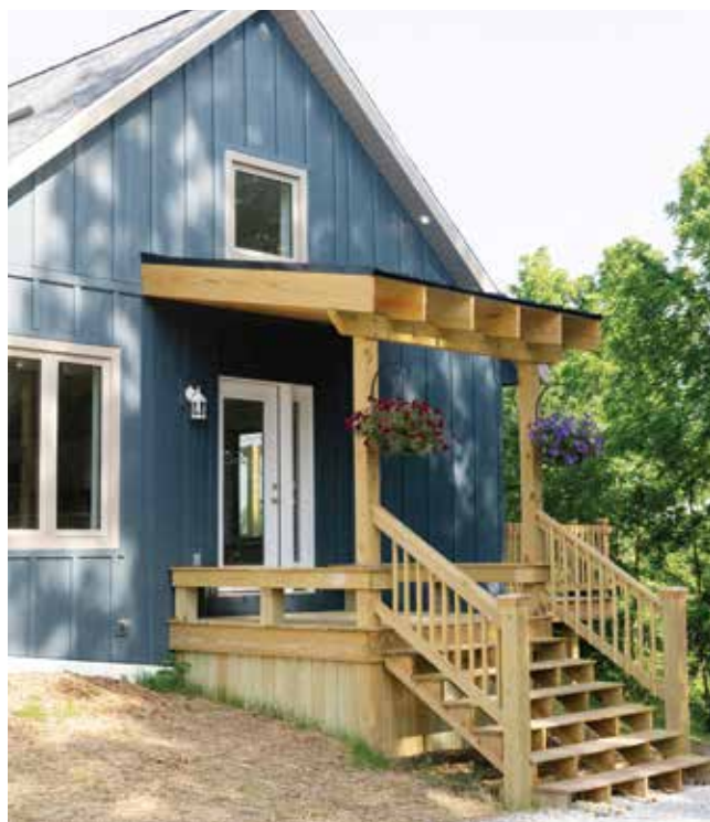
The affordable house prototype in Paoli was designed by Eskenazi students.
